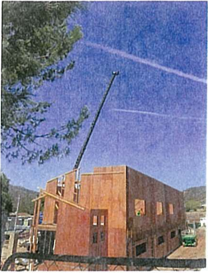
Construction sheeting July 14, 2015
