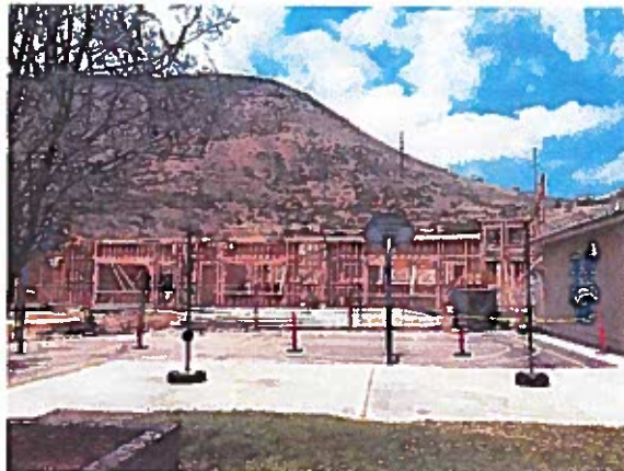
Construction Framing June 11, 2015
