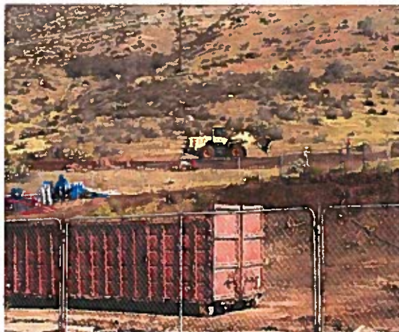
Construction Fencing & Grading March 19, 2015
