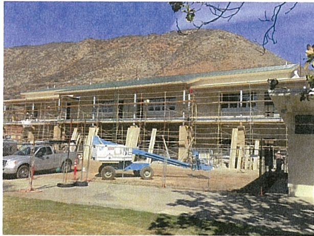
Roofing installation October 27, 2015
