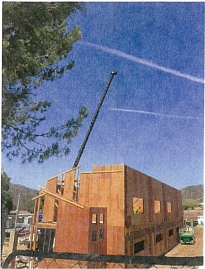
Construction sheathing July 14, 2015
