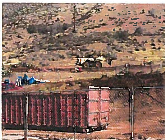
Construction Fencing & Grading March 19, 2015
